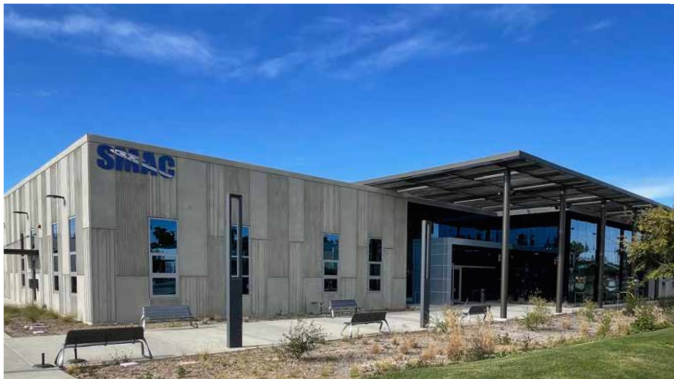
SMAC Corporate Headquarters and Factory
